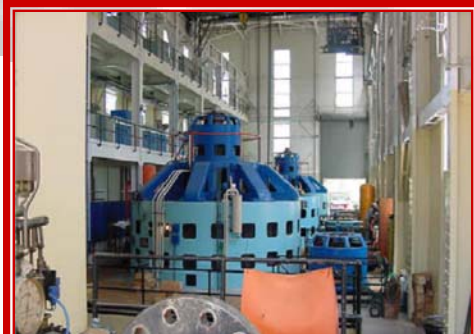
Oneida Powerhouse: (3) 14,500 KW GE Generators
